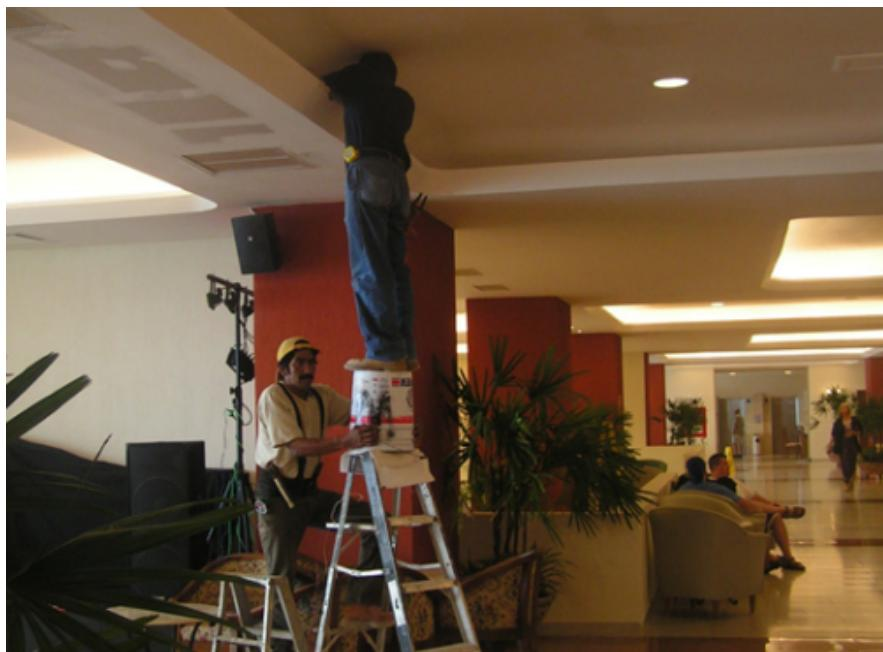
Most workers wouldn't dream of standing on the top cap of a stepladder, let alone the uppermost rung. But this worker is raising the stakes by standing on top of a bucket perched on the top cap. If this perilous setup started rocking, the worker holding the bucket would have little chance of preventing a serious fall. (Naval Safety Center)
