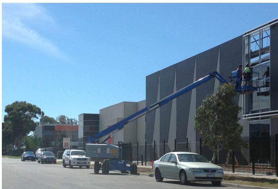
What's wrong with this picture? Actually, there are three things. First, the workers in the bucket are not wearing fall protection harnesses. Second, the counterweight on the lift is protruding into a traffic lane, with no traffic management practices in place, and third, there is no barricade to prevent people from walking under the boom or bucket. (Victorian WorkCover Authority, Australia)
