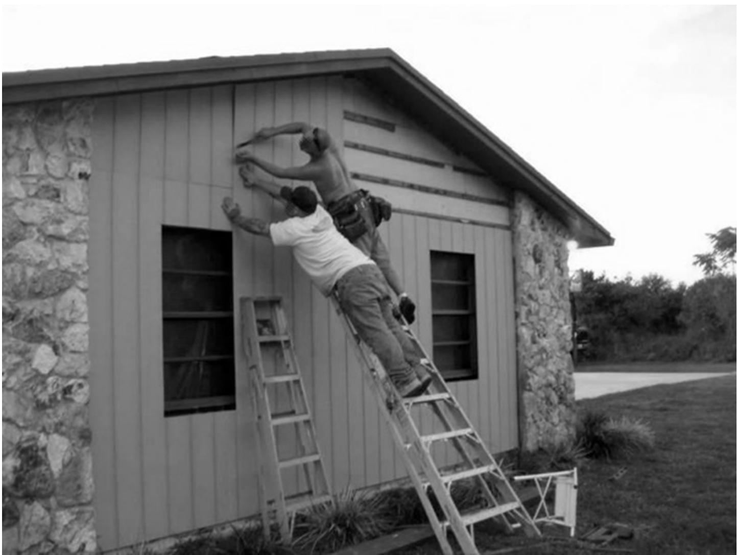
This image demonstrates a highly unsafe ladder use scenario. One worker is standing on top of a closed step ladder that is not fully opened or locked, while another person is dangerously climbing over him. Additionally, a second ladder nearby is not being used but is also positioned unsafely. These behaviors violate basic ladder safety rules and present a high risk of falls and serious injury.
