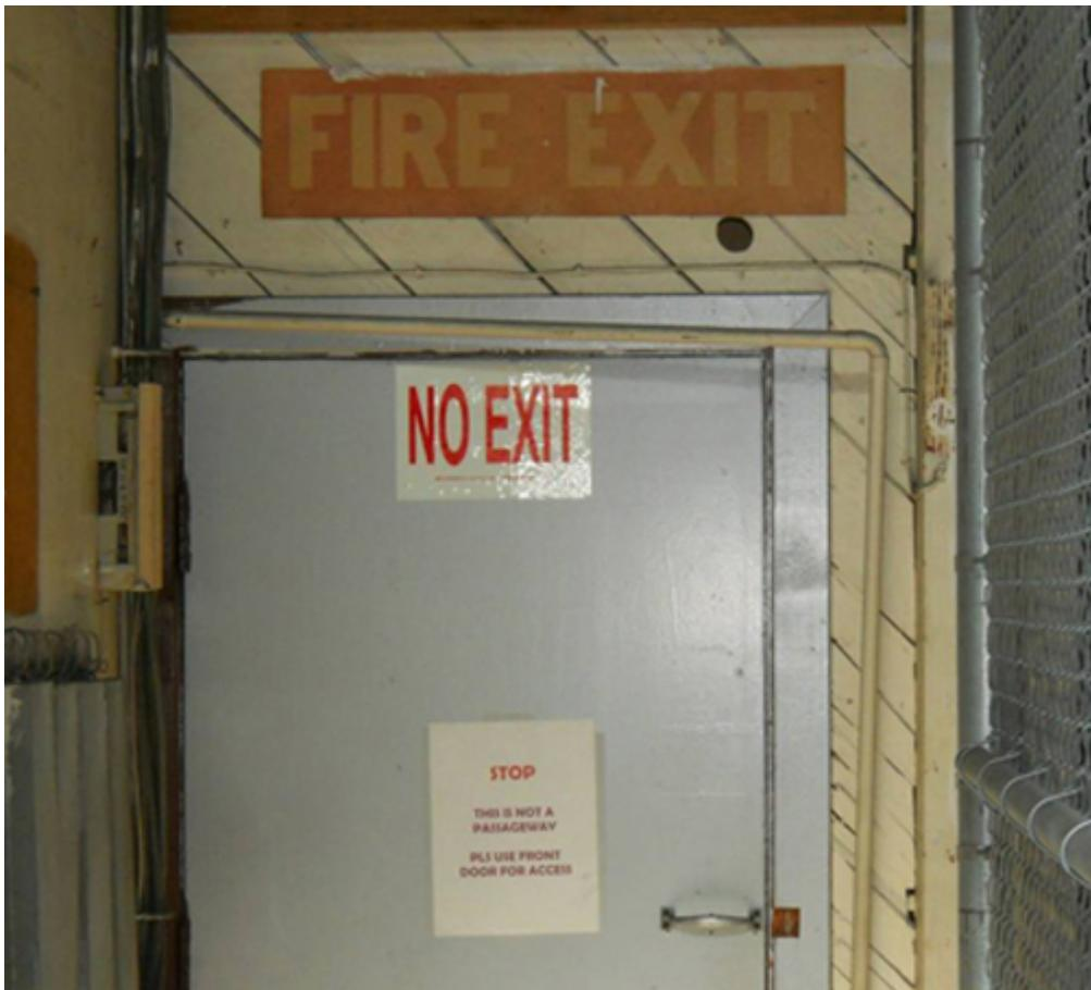
Make up your mind! Apparently, this door is NOT an exit. But the moment's confusion and hesitation that these mixed messages convey could prove deadly in a fire.
