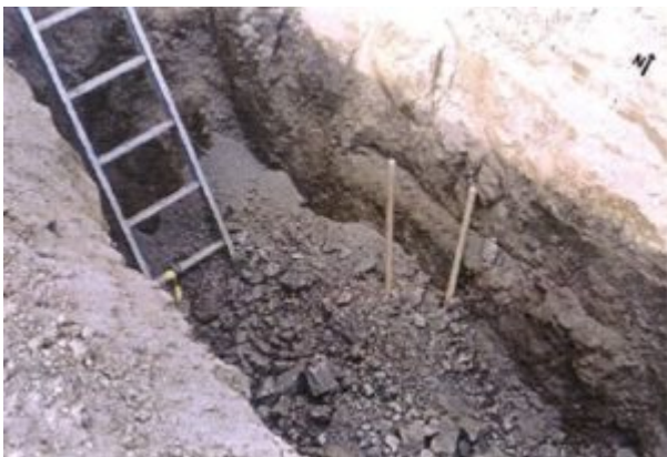
Figure 4. Incident Scene (The victim and his co-worker were buried near the west end of the trench.)
